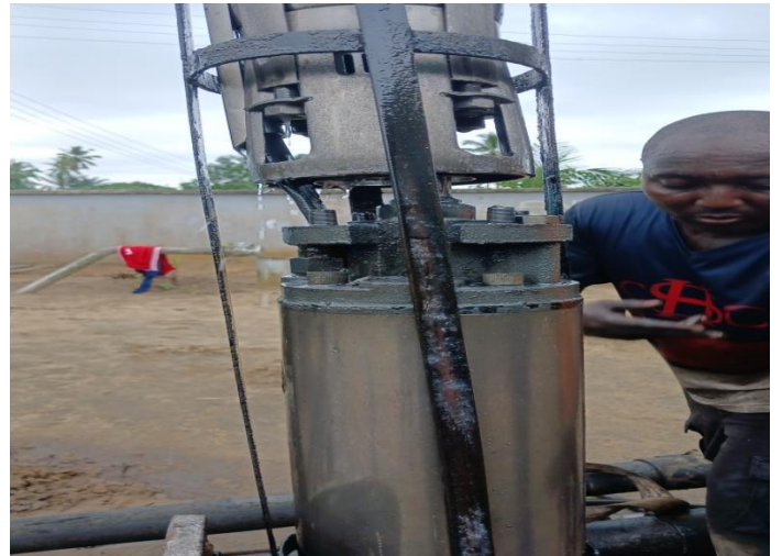
Pulling of defective pump from Borehole
