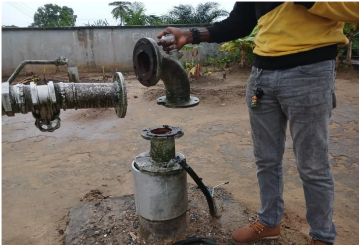
Pulling of defective pump from Borehole
