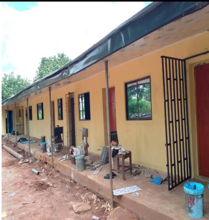
Painting of Office Building completed
