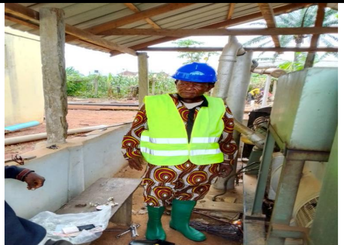
Overhauling of Generator set in Umunede
