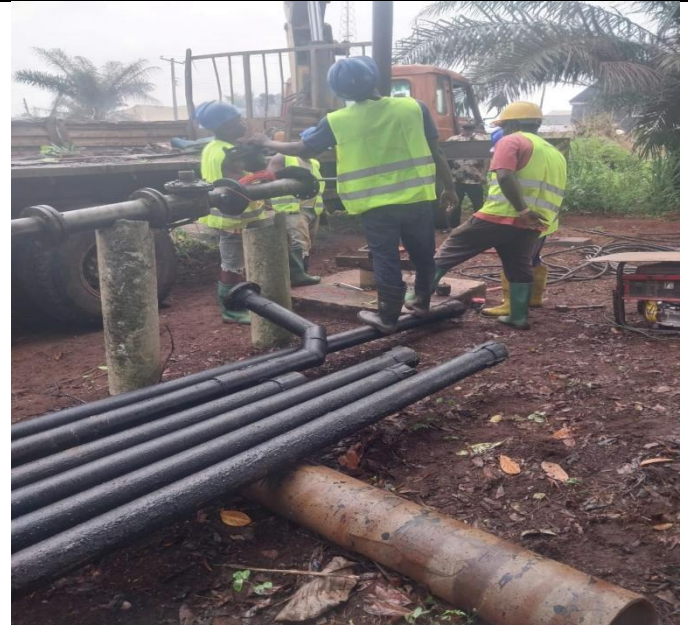
Installation of 25HP submersible pump in Umunede
