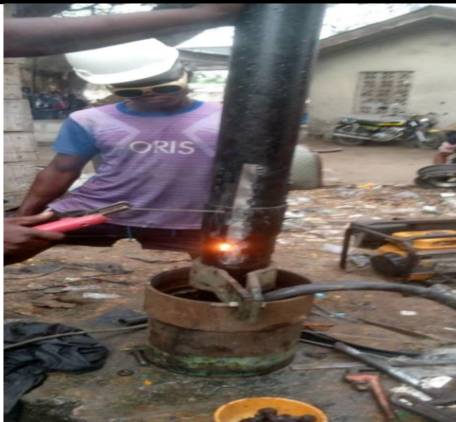
Submersible Pump Installation
