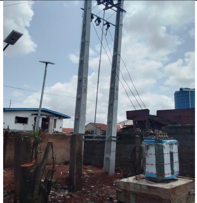
SIP Wire of the transformer was connected
