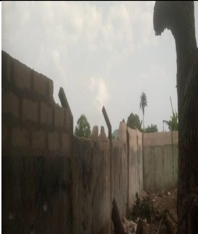
Increment in height of the existing block fence at the central headworks with two (2) additional blocks
