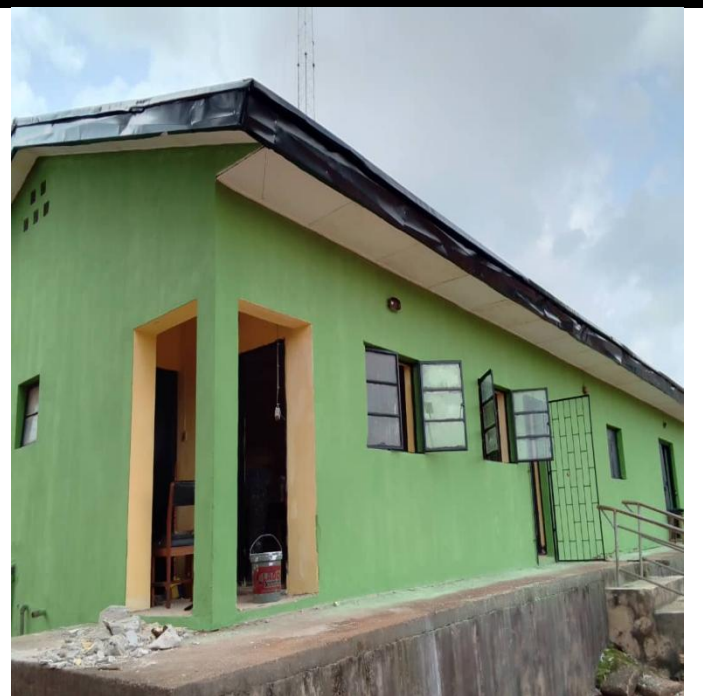
Rehabilitated Office Building
