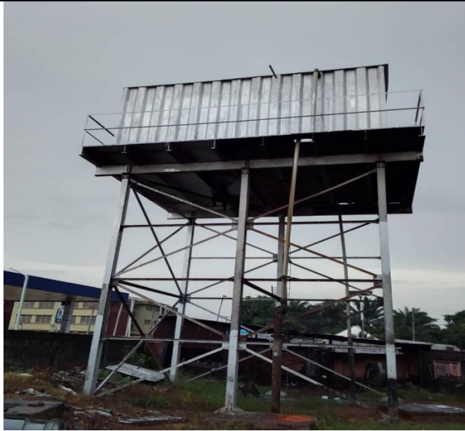
Washed and Painted 40,000 Gallon steel tank
