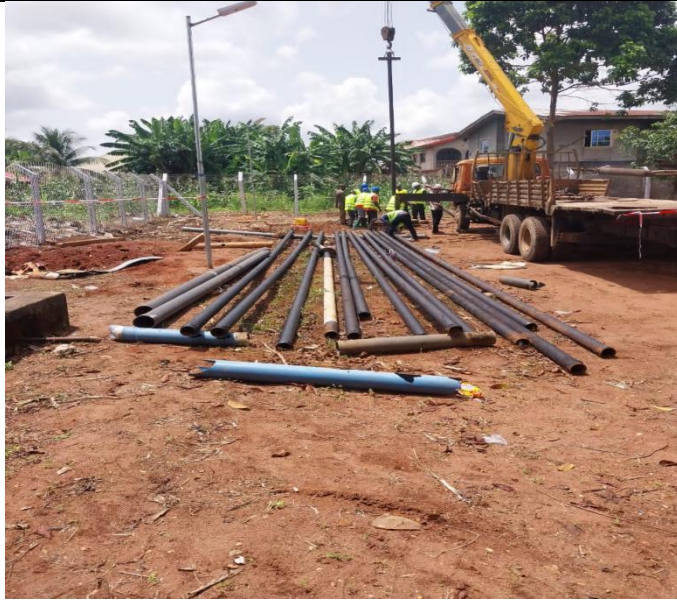
Pulling of 25HP Pump in Umunede
