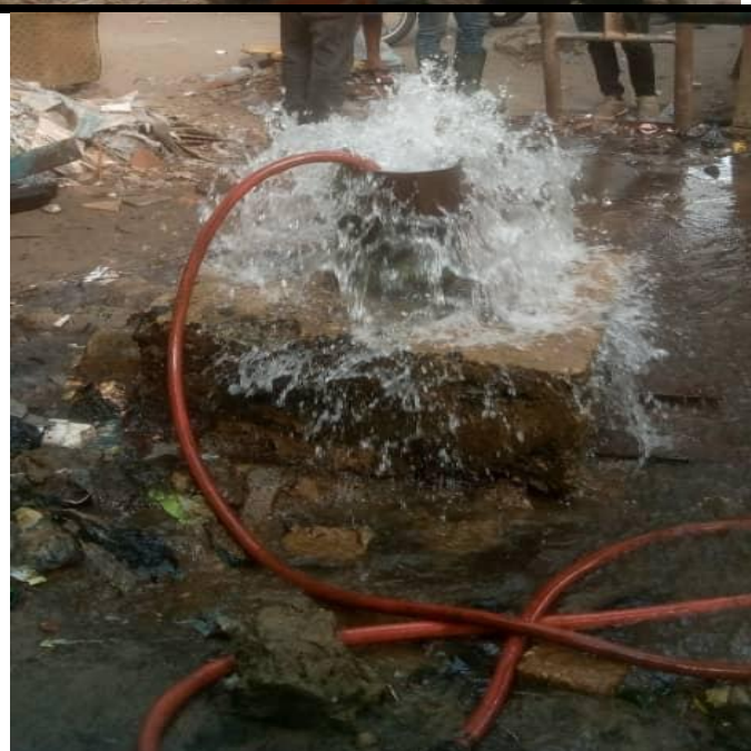
Re-Development of 250mm diameter borehole through airlifting by a compressor
