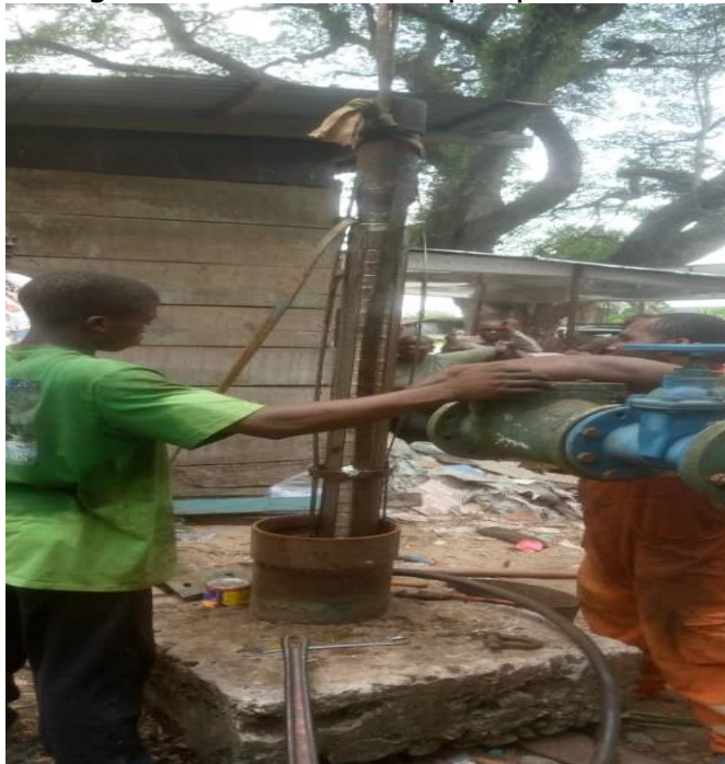
Pulling of 25HP submersible pump from borehole
