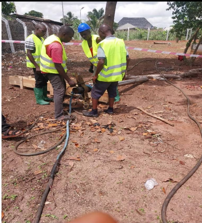
Installation of 25HP submersible pump in Umunede
