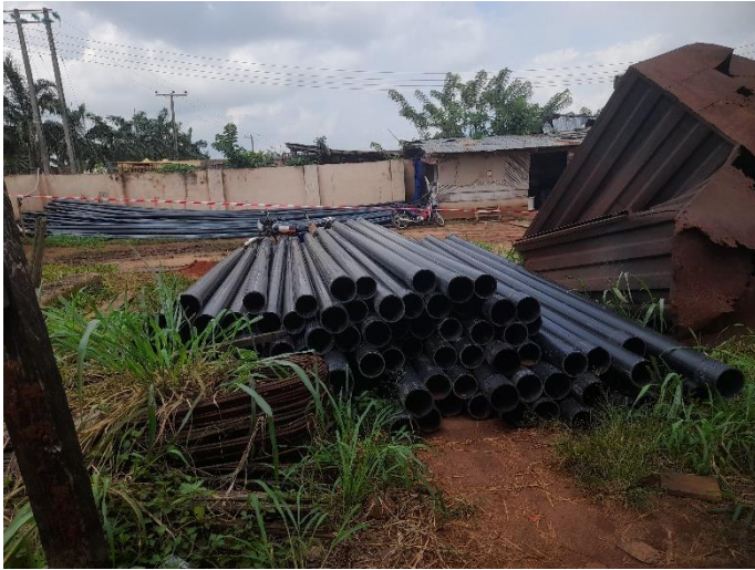
Delivery of 160mm UPVC and 110mm HDPE pipes @ Owa-Ekei
