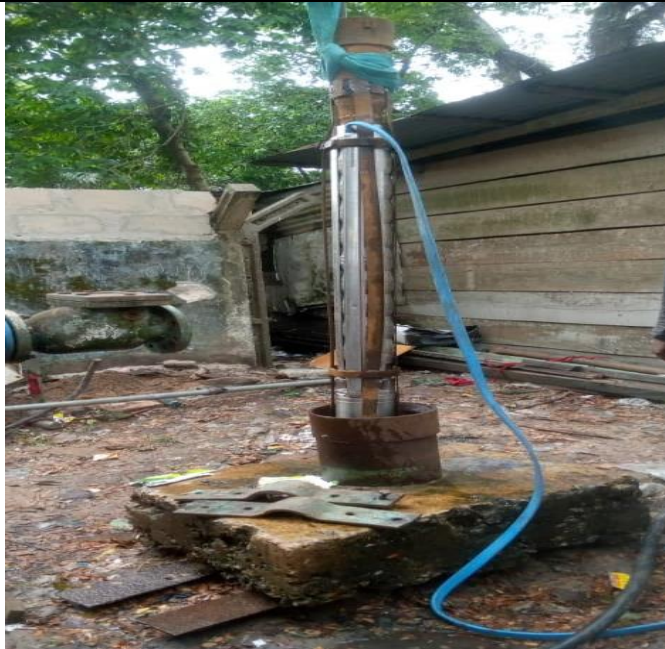
Submersible pump installation
