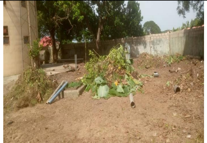
Clearing and Evacuating of Debris from site
