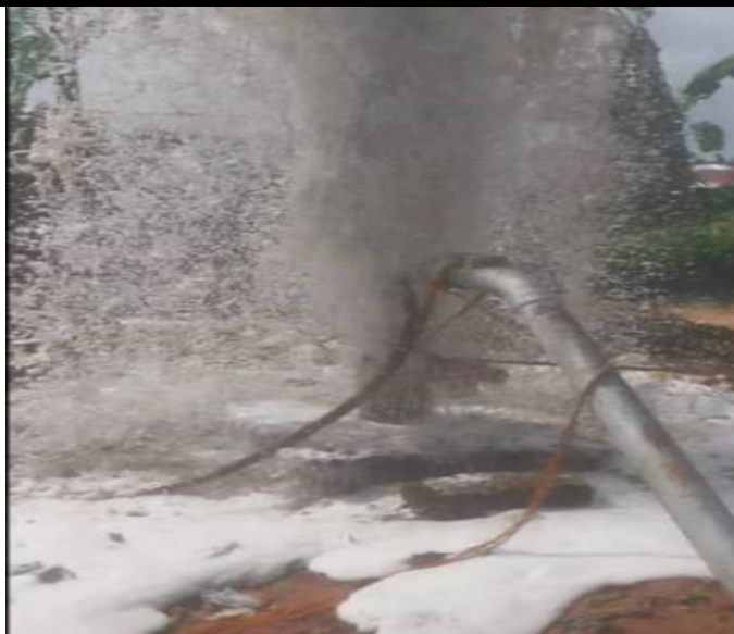
Working on Treatment Plant in Umunede
