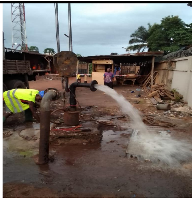
Testing of Water
