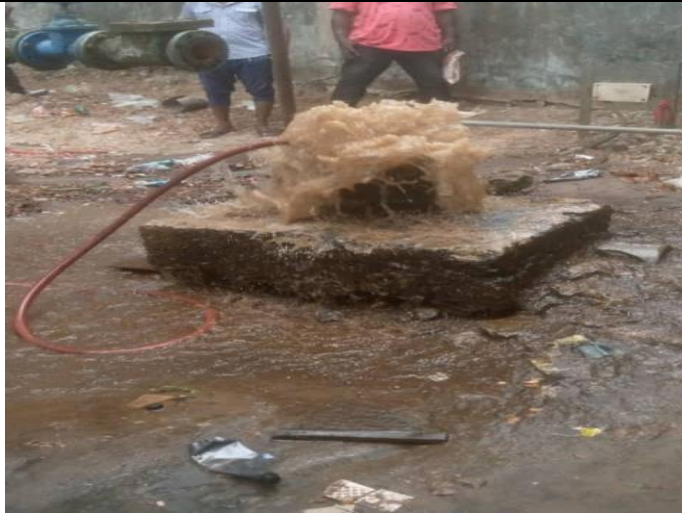
Re-Development of 250mm diameter borehole through airlifting by a compressor
