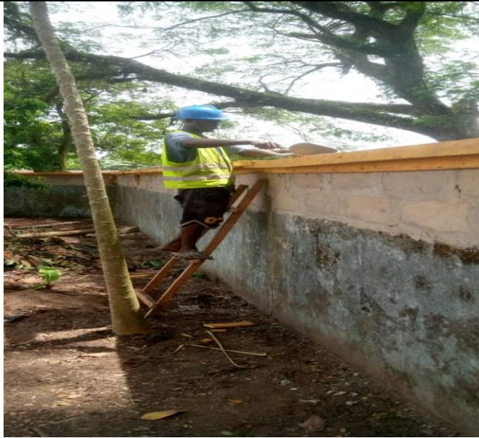
The copping of the block fence
