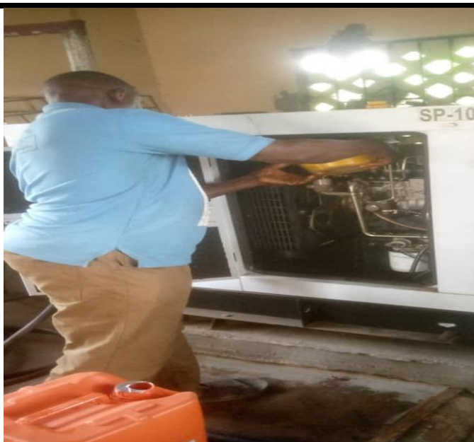
Overhauling of 100KVA Perkins generating set
