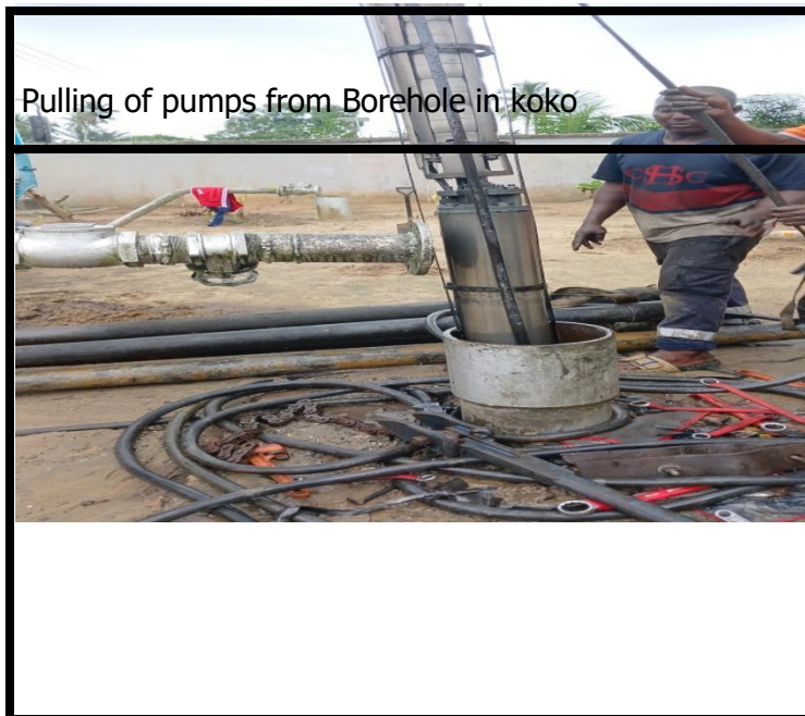
Pulling of Pumps from Borehole in Koko
