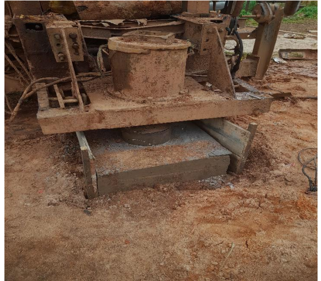
Drilling / Casing of 250mm diameter borehole @ Owa-Ekei
