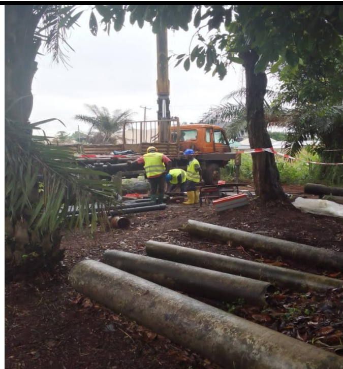
Development of Borehole with air lift Compressor
