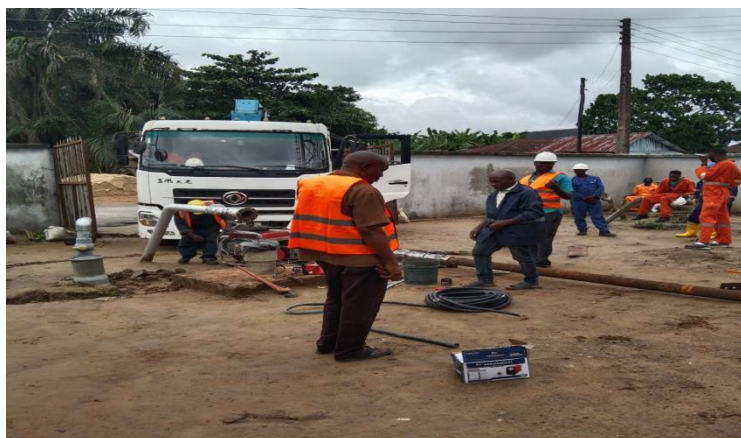
PREPARATION FOR THE INSTALLATION OF 25HP PUMP BY DESUWACO AND CONTRACTORS' TEAM
