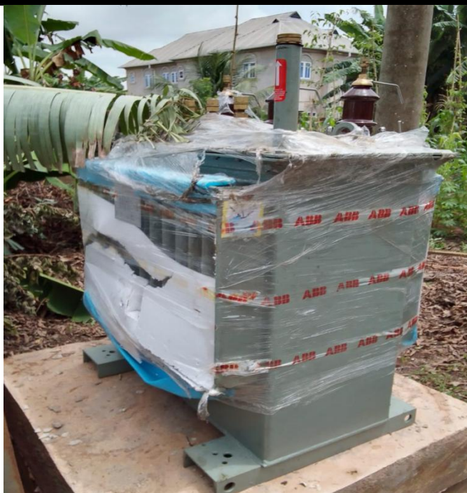
Installation of 200KVA Transformer
